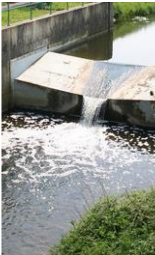
Stream Gauge Measurement
