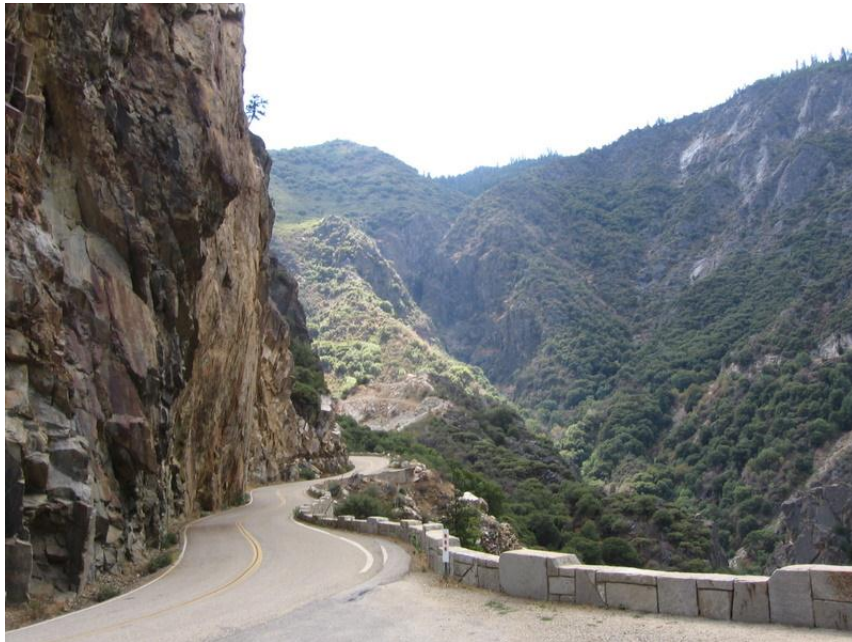
Figure 2. Cliff-side road in Kings Canyon.
