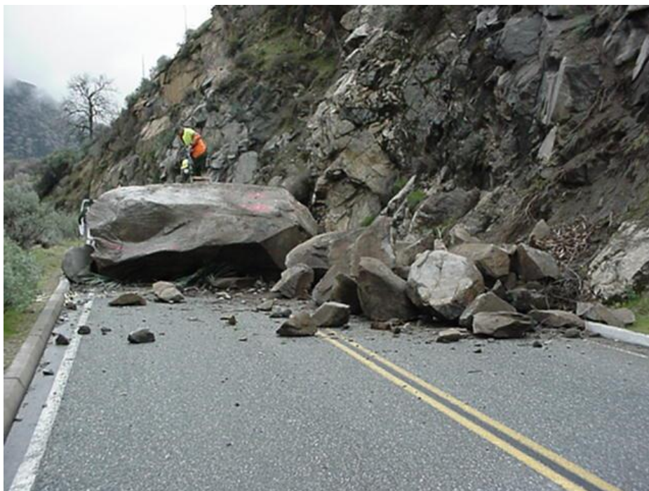
Figure 1. Rock fall about a mile below Tunnel Rock, January 28 2005.
