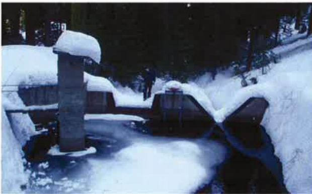
Figure 2. One watershed in the Teakettle Experimental Forest is used as a control watershed; it has never been disturbed by roads or timber harvests. This photo shows the Teakettle stream at the Bull Site in winter; the weir and basin were constructed in the 1940s, and retrofitted with modern instruments for KREW measurements. Photo: S. Eagan
